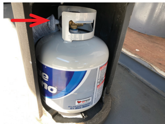
Find valve at top of tank
